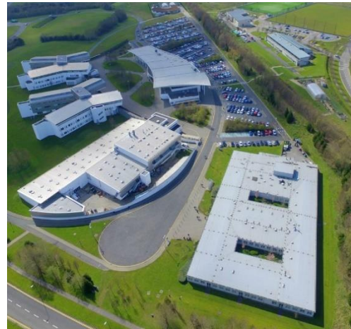
FIGURE 3.3: AERIAL VIEW OF IT BLANCHARDSTOWN
